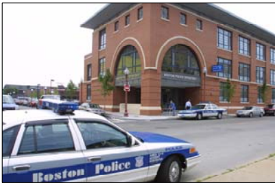
Area D-4 Police Station
