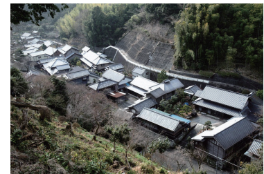
Preservation Districts for Groups of Traditional Buildings of Hanazawa, Yaizu City (Shizuoka Pref.), assigned in September 18, 2014
