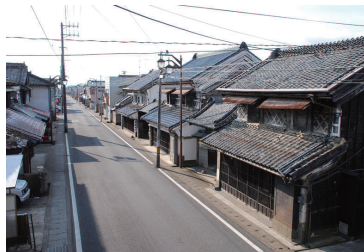
Preservation Districts for Groups of Traditional Buildings of Murata, Murata Town (Miyagi Pref.), assigned in September 18, 2014
