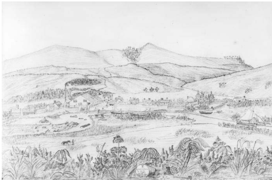
Fig. 13: Thomas Reid Sawmill and settlement, Coromandel, Auckland, New Zealand 1866 Alexander Turnbull Library B-038-011
