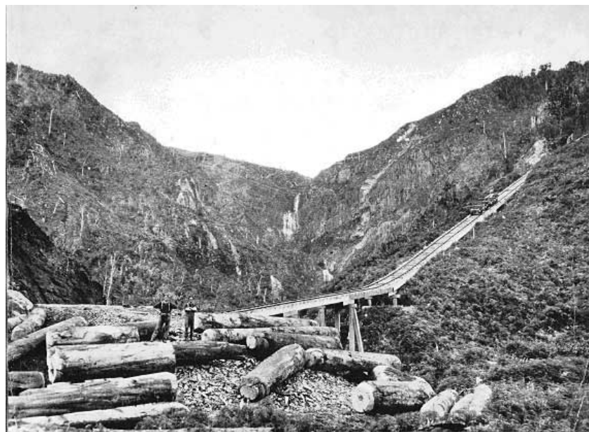
Fig. 14: 'View of Billygoat Landing, with empty bogeys being winched up the incline. Billygoat Falls are near the centre and smoke from the steam winch boiler can be seen towards the top right.' www.thetreasury.org.nz/
