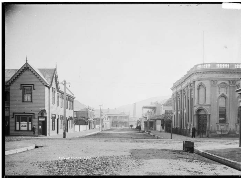
Fig. 12: Bank of New Zealand, corner of Brown and Albert Streets, Thames, circa 1900, seen here on the right across the road from the Wharf Hotel. Price Collection, Alexander Turnbull Library 1/2-001554-G
