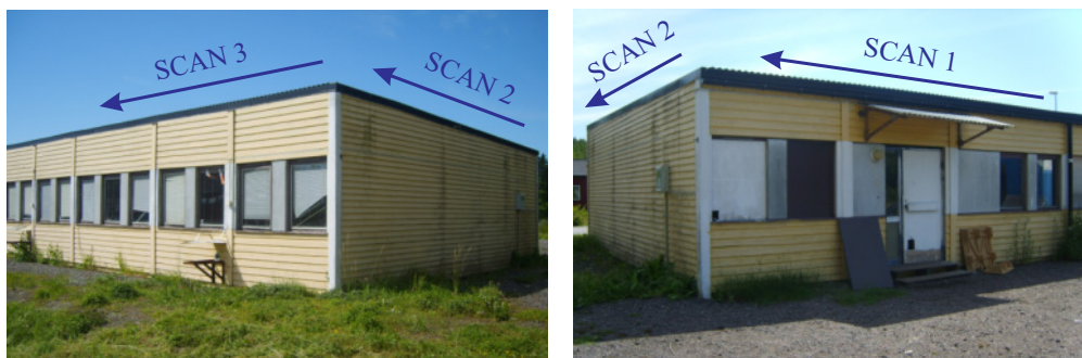
Fig. 4.3.6: Photos of scanned building. Stockholm Rescue Center - Sweden.
