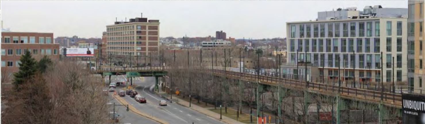
View from the south from the Museum of Science parking garage
