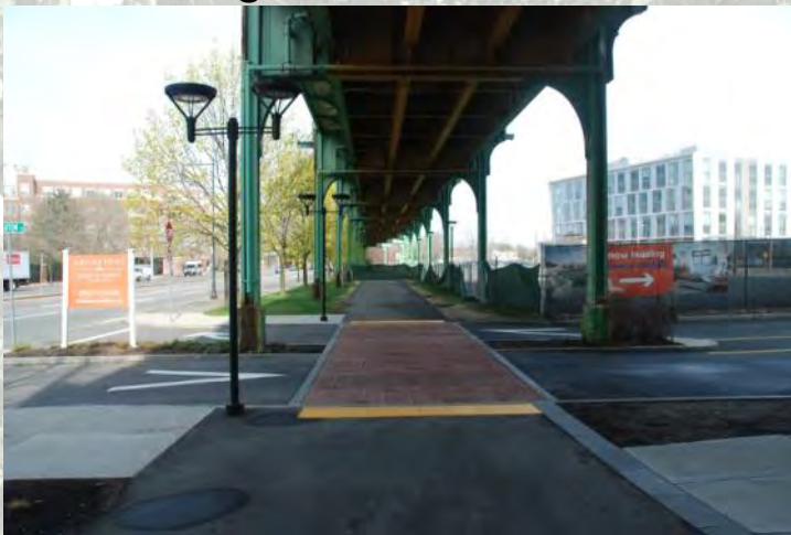
View beneath existing viaduct
