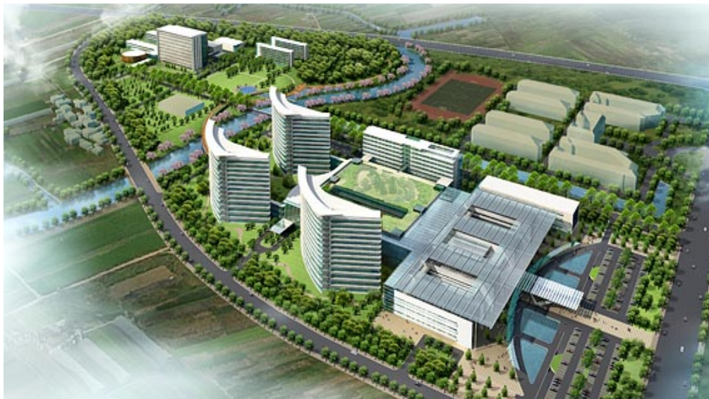
Rendering: Shanghai Eastern Hepatobiliary Hospital Anting Campus 107 (completed in Oct. 2015 containing 1,500 beds) 108
