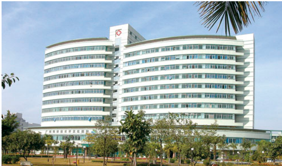
Guangzhou Economic and Technology Development Zone Hospital 1349
