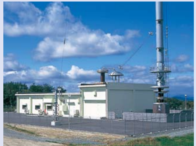
▲Standard time and frequency transmission station
