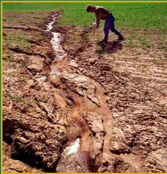
Damage of work due to excessive rainfall
