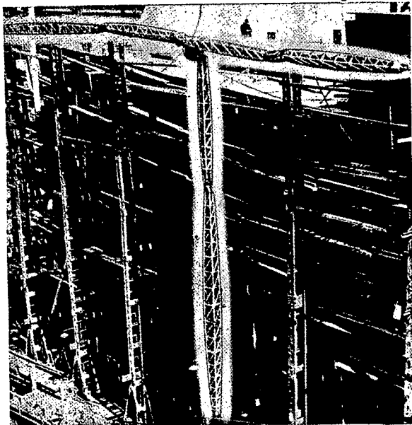
Fig. 1. — A tree grows at Kearny up a staging tower. Horizontal branches, left and right, are seen at the top
