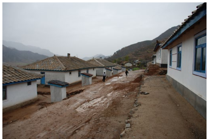
These government built houses in South Pyongan province have been erected on higher ground to house families who lost their homes during the flash floods in July 2012. Series North Korea: Daily life remains a struggle (2012) © European Commission DG ECHO
