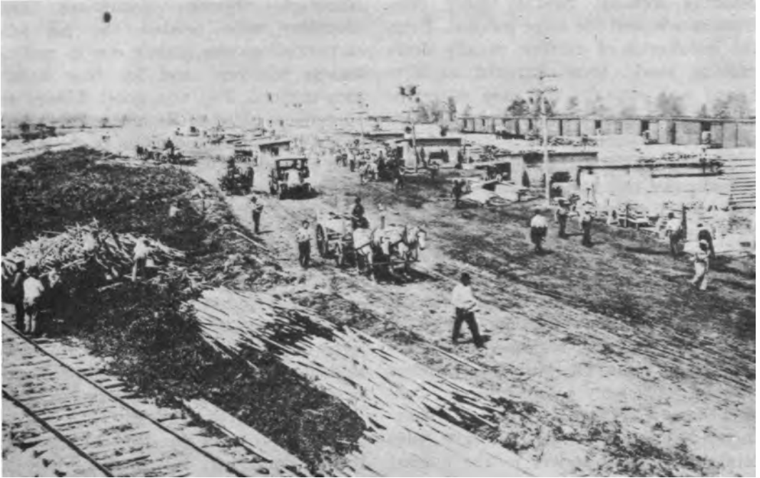
CAMP CUSTER, MICHIGAN, UNDER CONSTRUCTION, 1917
