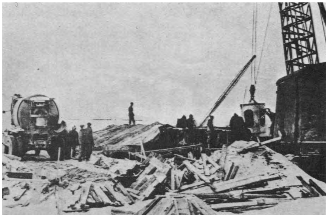
POURING CONCRETE IN SUBZERO WEATHER, PINE CAMP, NEW YORK
