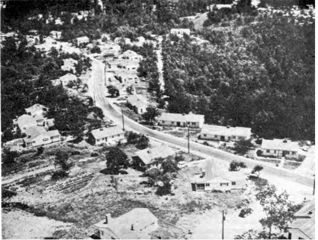
CEMESTO HOUSES ON BLACK OAK RIDGE, Clinton Engineer Works, Tennessee.
