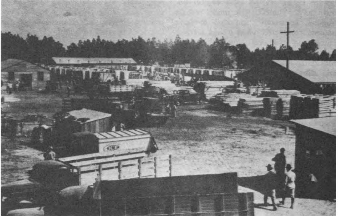
PREFABRICATING YARD AND SAWMILL, CAMP BLANDING, FLORIDA
