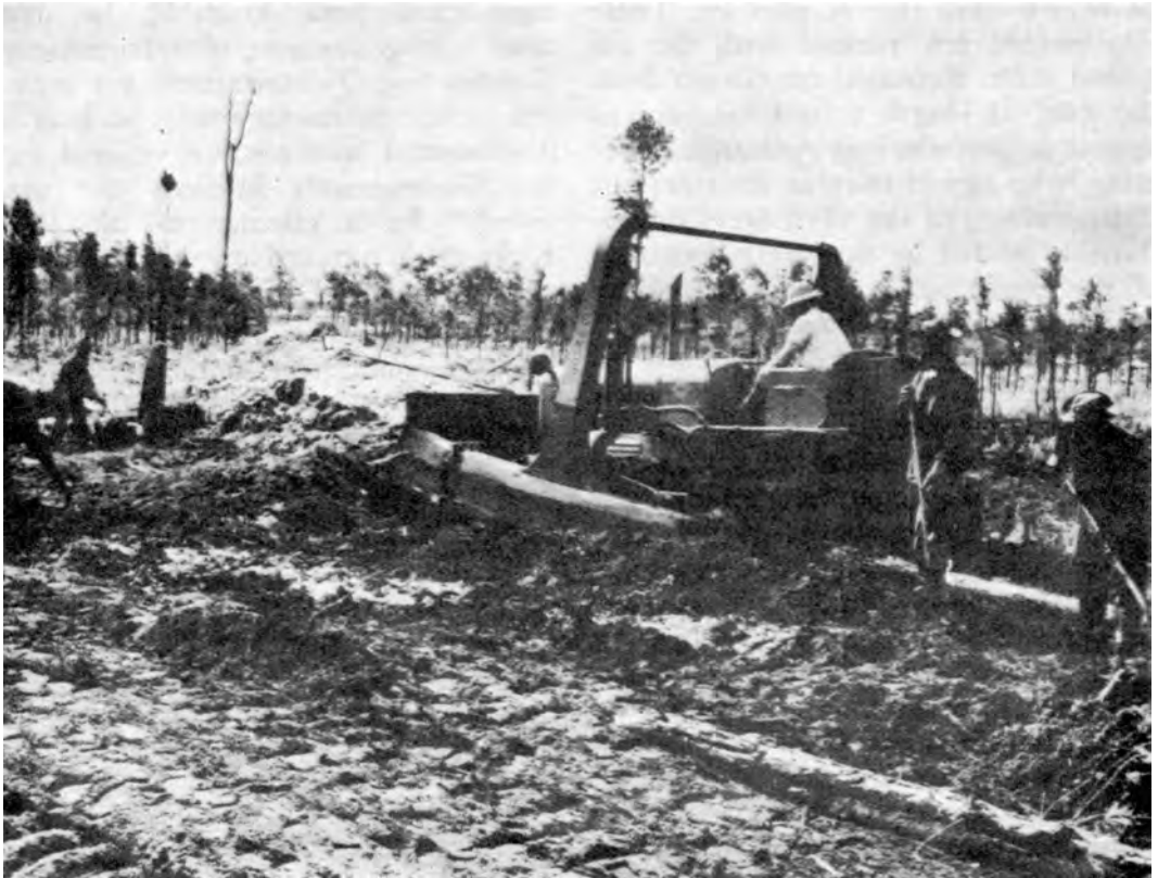
CLEARING SWAMPS AT CAMP BLANDING, FLORIDA
