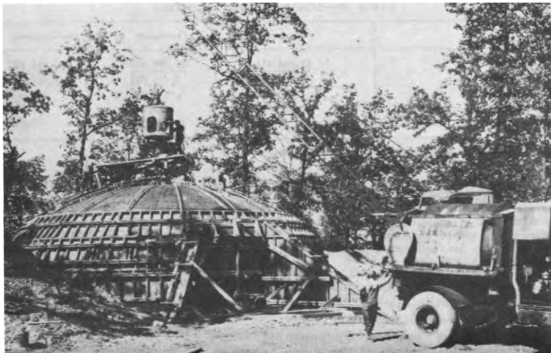
CORBETTA BEEHIVE MAGAZINE UNDER CONSTRUCTION
