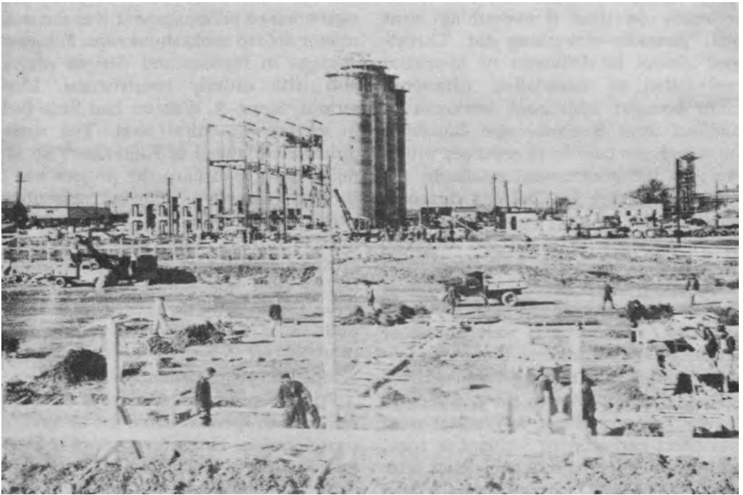
CONSTRUCTION UNDER WAY AT INDIANA ORDNANCE WORKS, 1940.
