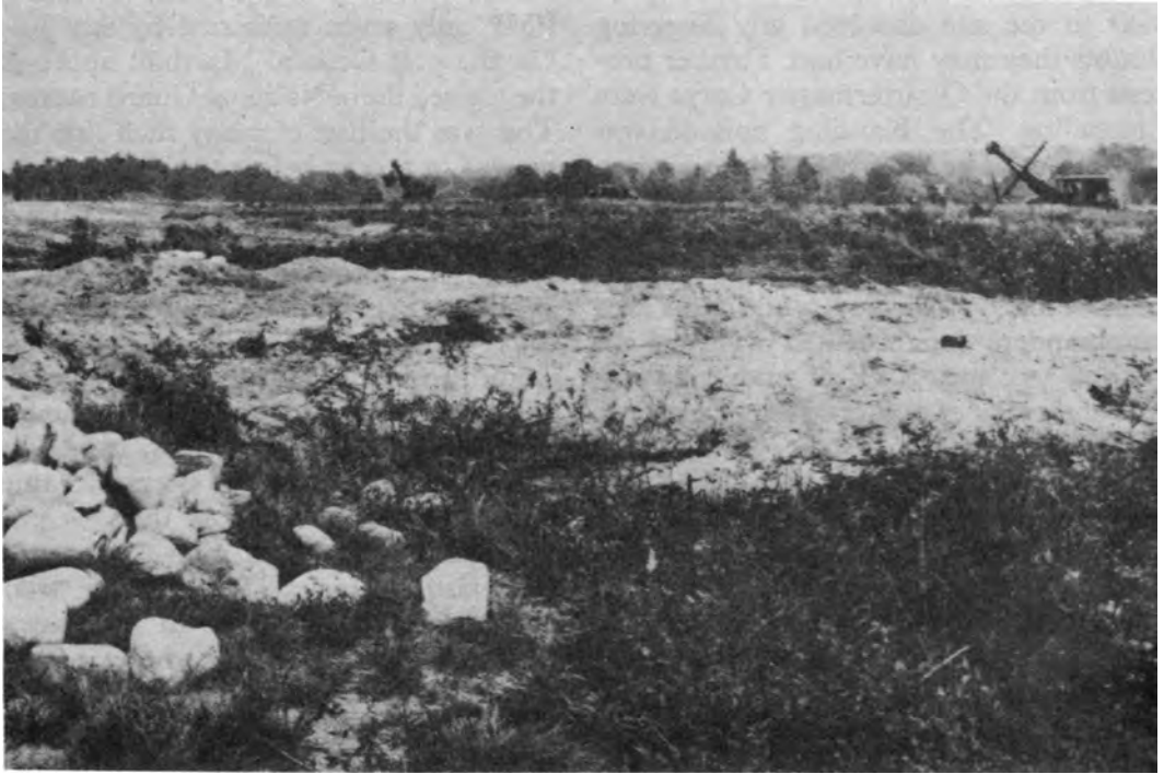
EXCAVATION AT FORT DEVENS, MASSACHUSETTS
