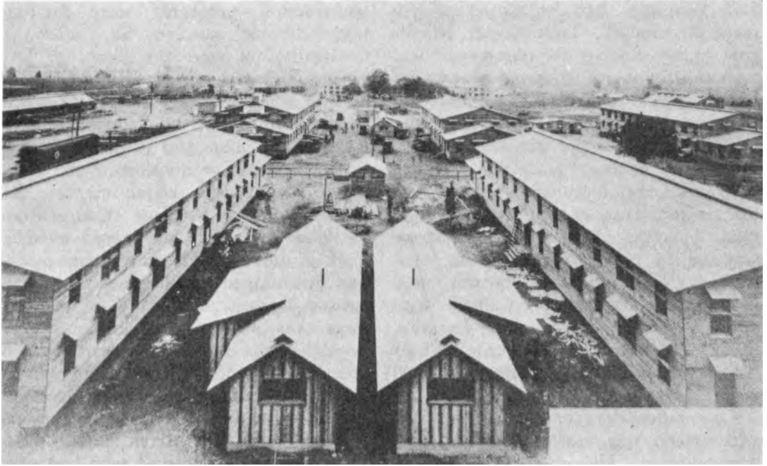
BARRACKS AND LAVATORIES, CAMP DIX, NEW JERSEY
