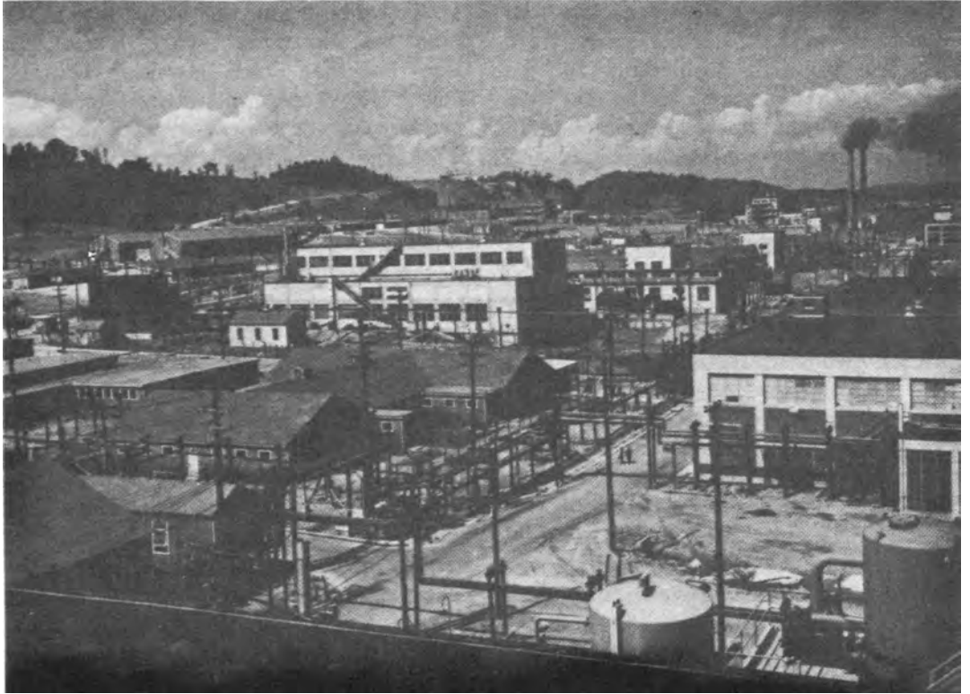
Y-12, ELECTROMAGNETIC PROCESS PLANT
