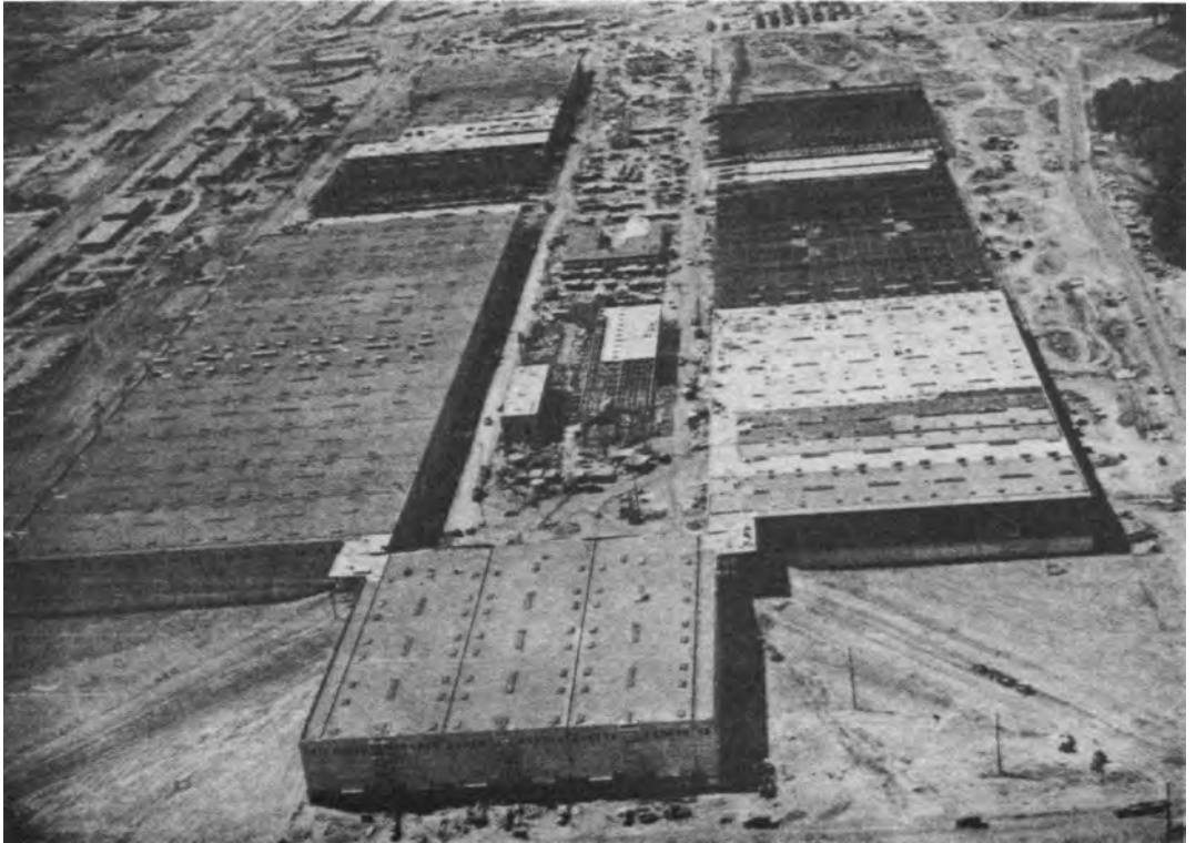
K-25, GASEOUS DIFFUSION PLANT NEARING COMPLETION
