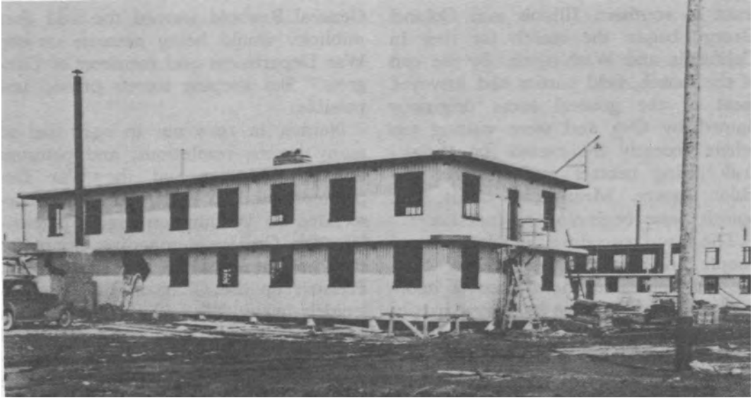
EXPERIMENTAL STEEL BARRACKS
