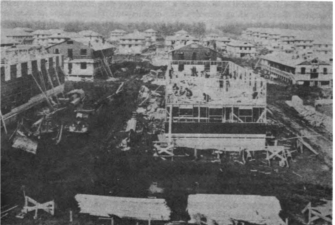
BUILDING BARRACKS, CAMP LEONARD WOOD, MISSOURI
