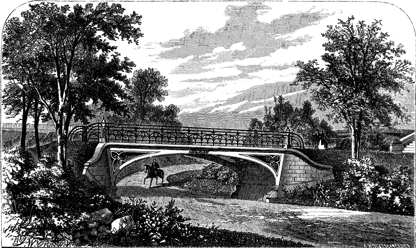
ARCHWAY OVER BRIDLE ROAD NEAR SOUTH GATE HOUSE OF CROTON RESERVOIR.
