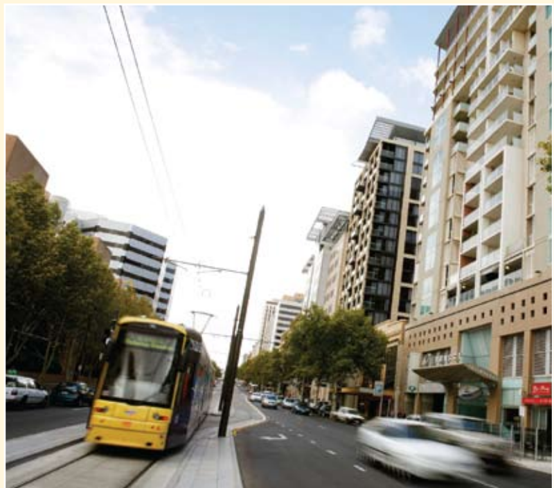
The tramline extension, North Terrace
