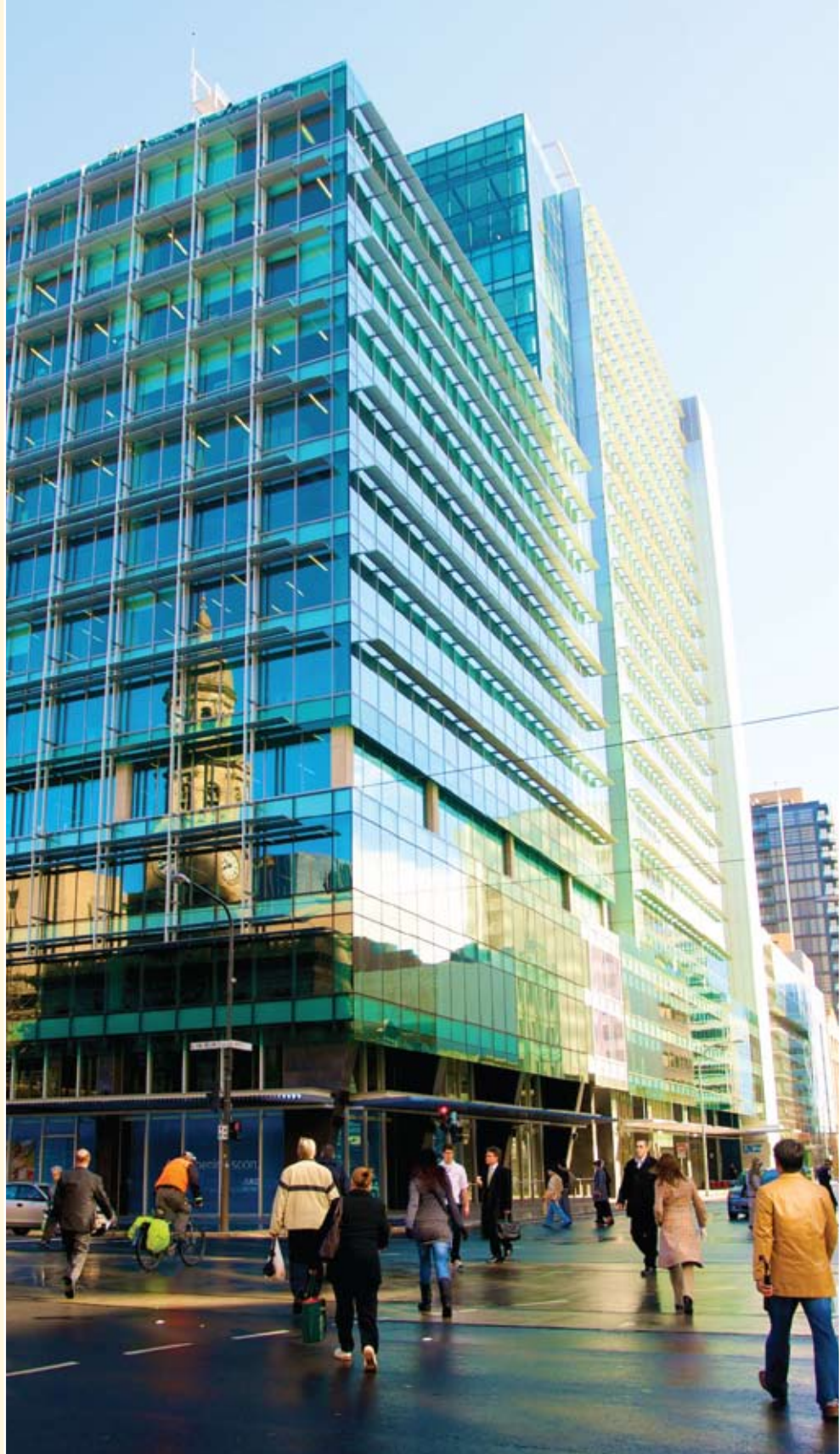
Tower 2, Ernst & Young Building
