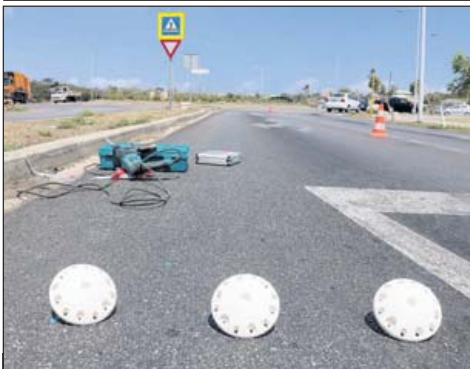
Curaçao's Public Works Department is having plastic objects installed in the road surface at the approaches to several roundabouts on the island, warning motorists to slow down. Along with clearly visible maximum speed traffic signs, the move is to help prevent damage to cars and so-called street furniture alike.
