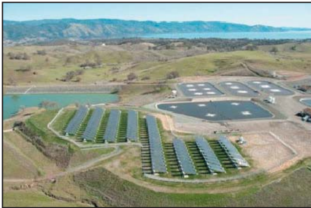
Northern California Power Agency's solar array. Photo by S. Eneby.
