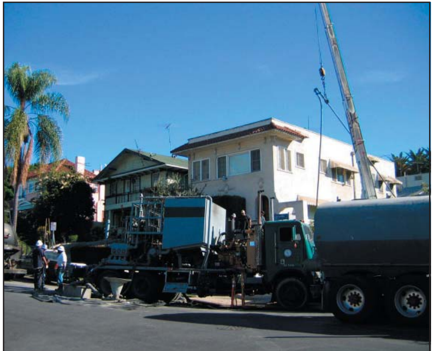
Photo 6. Well L.A.R.R. Co. 1A. Cementing equipment is positioned to plug the well with cement. Photo by G. Brandt.
