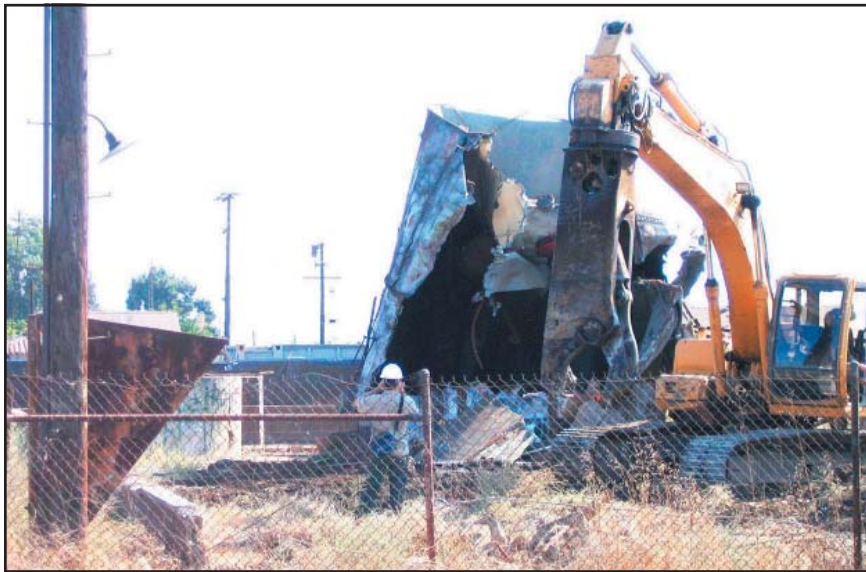
Photo 3. Tank farm behind preschool being demolished. Photo by C. McCullough.
