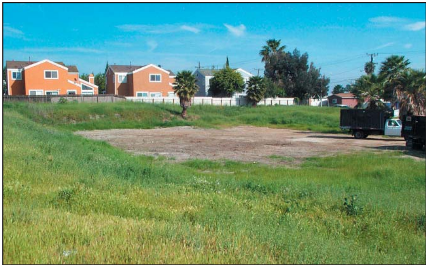
Photo 2. Howard Community tank farm after demolition. Photo by M. Johnson.
