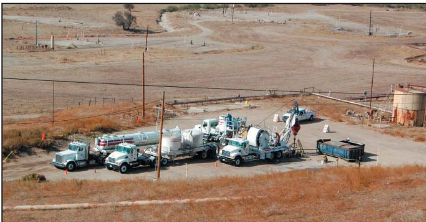
Photo 5. Chevron USA Inc. plugged and abandoned long-term idle wells on the "WP Hammon Fee B (NCT-2)," "WH-RF," "Williams Holding," and "GWP" leases. Photo by R. Brunetti.
