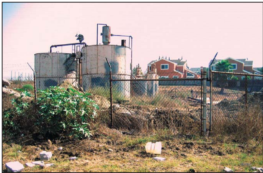
Photo 1. Howard Community tank farm prior to demolition. Photo by N. Saito.
