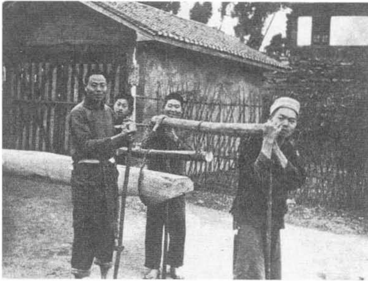
Fig. 279. Distribution of load among many porters, an ancient Chinese method still commonly used (photo. Gordon Sanders, near Chungking, 1943).
