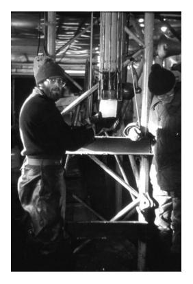
Fig. 14. One of the first cores recovered by TELGA-14M thermal drill in hole No. 5G.
