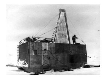
Fig. 8. The mobile drilling shelter PBU-2 towed to Vostok (summer season of 25th SAE, 1980).
