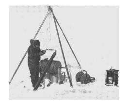
Fig. 2. First experience of thermal drilling at Vostok station during the 4th CAE (from Ignatov, 1962).
