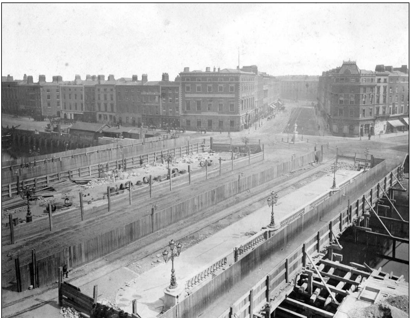
Fig. 8. O'Connell Bridge (under construction) 1879
