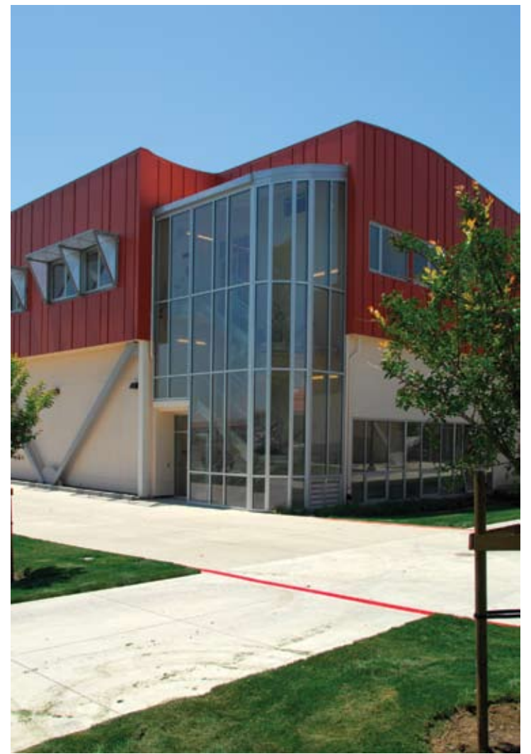
The Barbara Mertes Center for the Arts at Las Positas College opened in August. Incorporated within the facility is a 550 seat theater and a 175 seat black box theater. A 1500 seat amphitheater is situated outdoors. In the backstage area are several technical theater rooms, a scene shop, a costume shop, storage for scenery and props, and a formal green room. There is a 800 square foot gallery, the first formal art gallery on the campus. There is a two story high grand lobby with an atrium.
