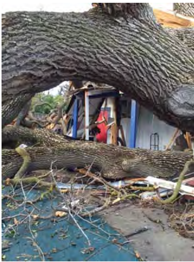
A 400-year-old Valley Oak, the largest in the area, fell on the morning of Feb. 9, the day after construction took place at the Sunset Cabana Club Pool building. The ancient tree had been healthy; it fully leafed in each year, and cross-sections taken while removing the fallen trunk showed that it was sound.
