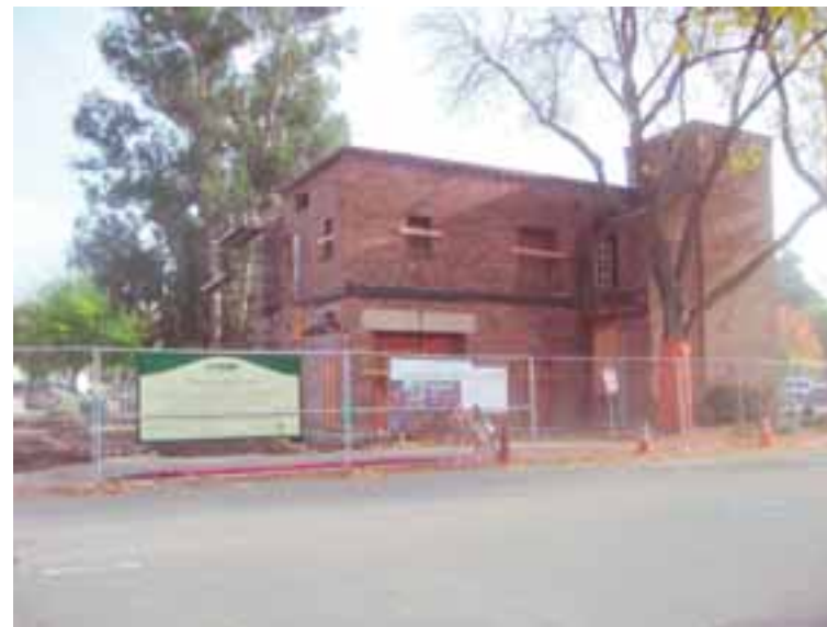
Work is underway on the Firehouse Arts Center in downtown Pleasanton.
