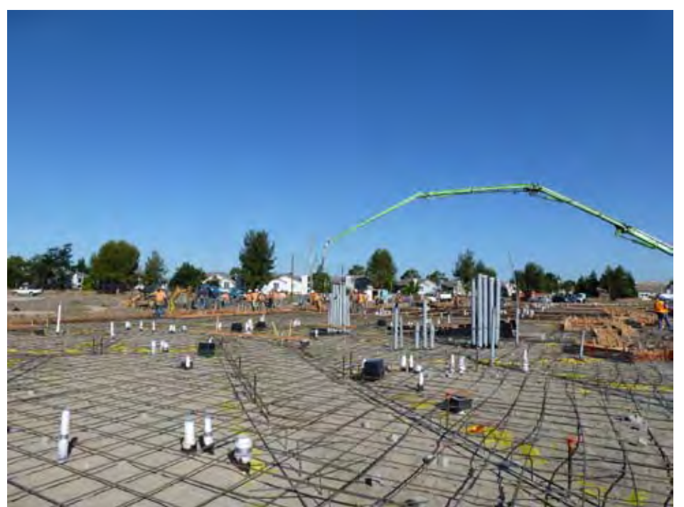
Work is underway at the new retirement community in Pleasanton.
