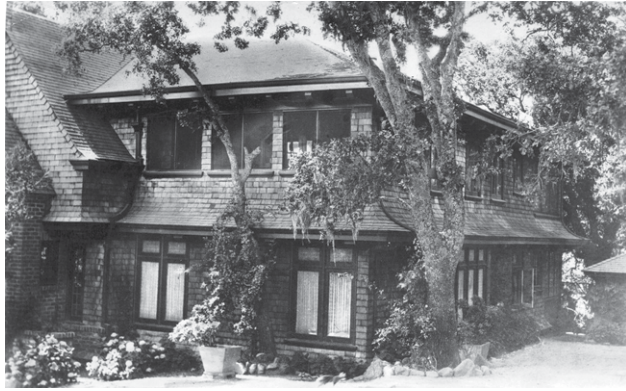
Pictured is the Ogeedankee house.
