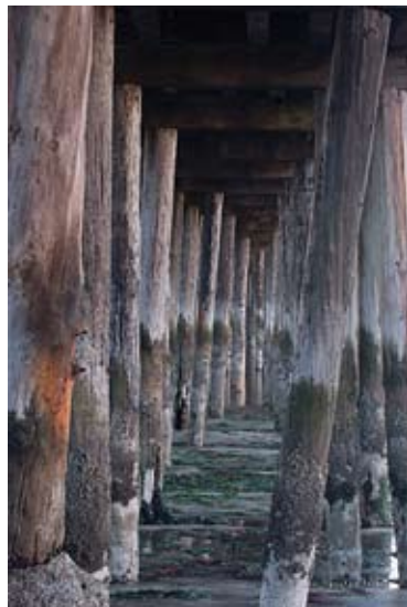
"Pilings" is an example of Puspha's work.
