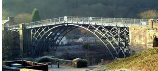
1779 - The world's first cast iron bridge is built. The Iron Bridge spans 100ft (30m) over the River Severn at Coalbrookdale (UK).
