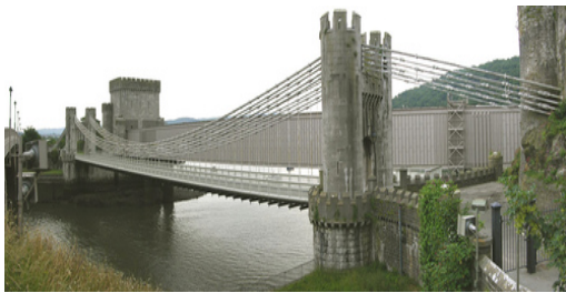
1826 - One of the world's first road suspension bridges, Cowny Suspension Bridge , spans across Cowny River, Wales.
