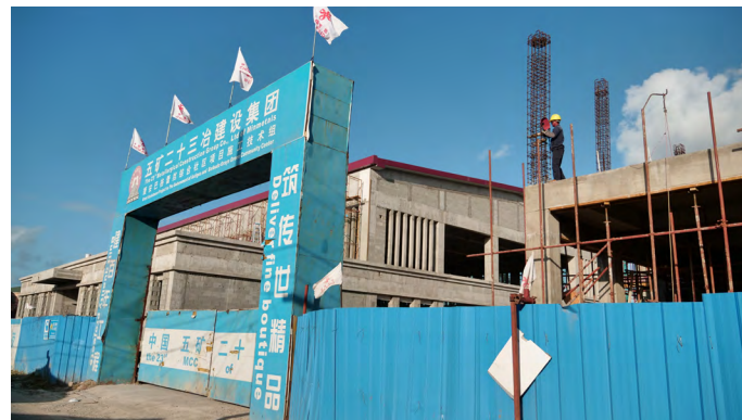
(Knuckle Block Under Construction)
