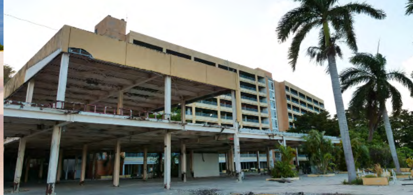
(Royal Antigua Hotel under construction)
