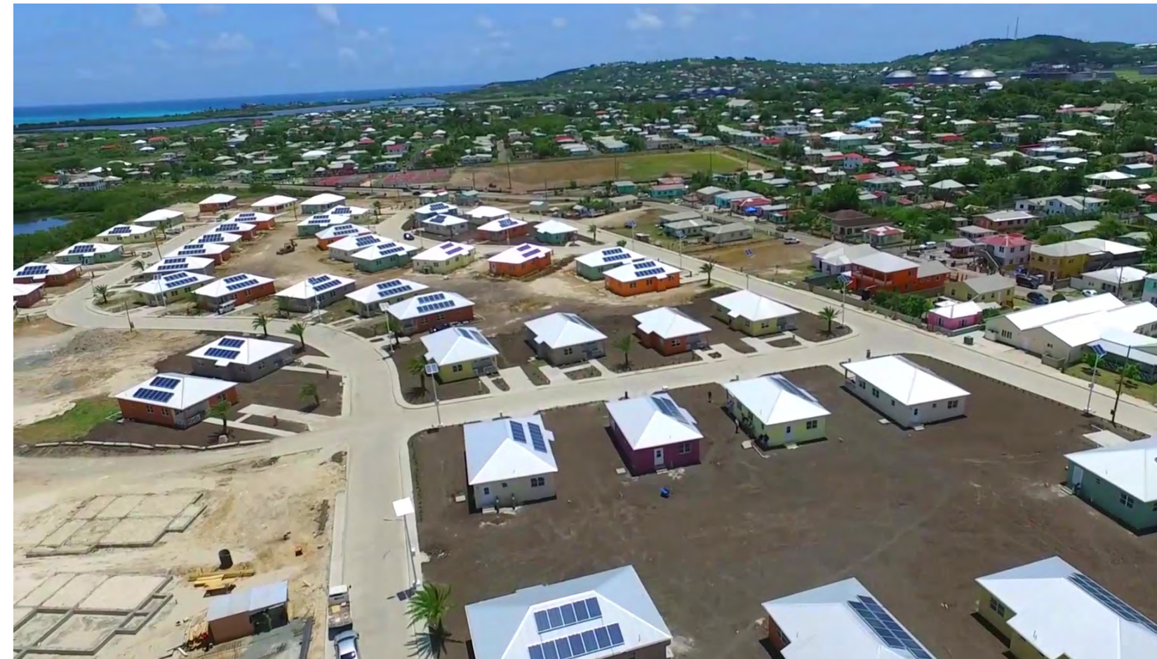
Housing at Dredge Bay
