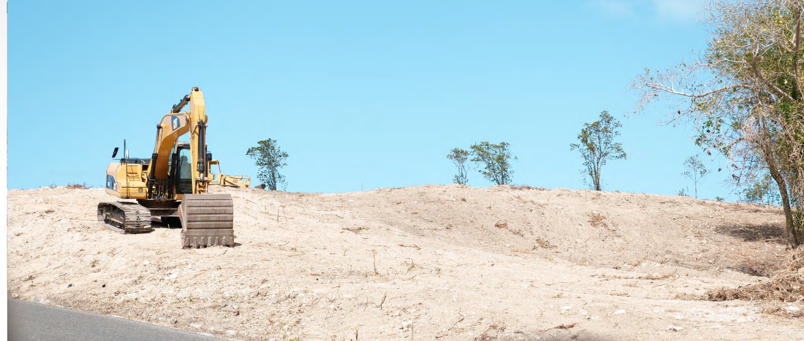
(Land clearance for distribution at Friar's Hill)
