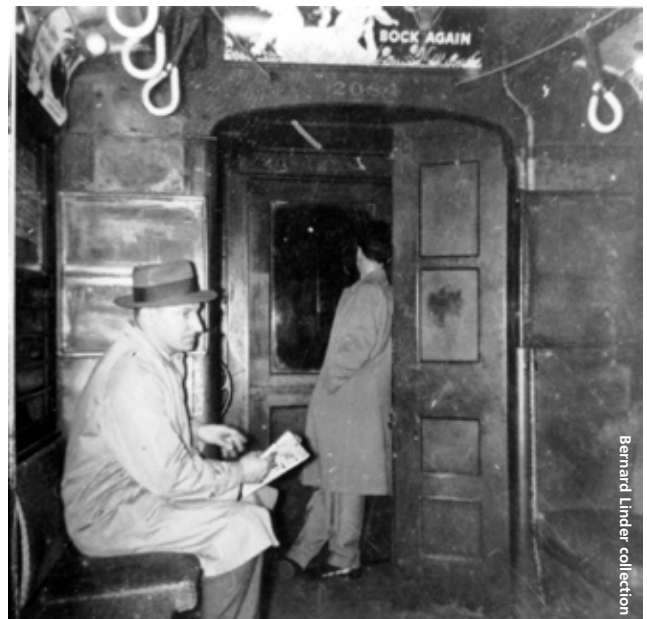
Interior of composite car 2084 — the Motorman's cab and front window have been rebuilt for elevated service.
