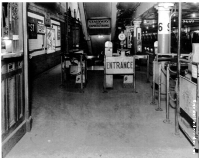
The 96 th Street-Broadway station. On the left is an agent's booth and on the right is a door that could be unlocked by the agent when an employee wanted to enter. This door was installed about 1936 to reduce fare evasion. It replaced chains that were opened by employees entering the station.
