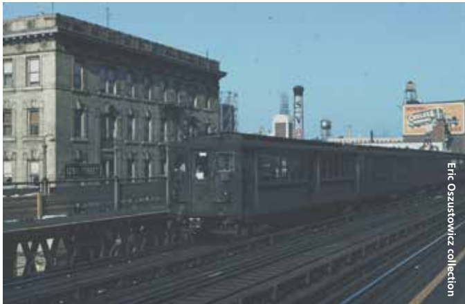
Deck roof Hi-Vs on the Broadway Line at 125 th Street.
