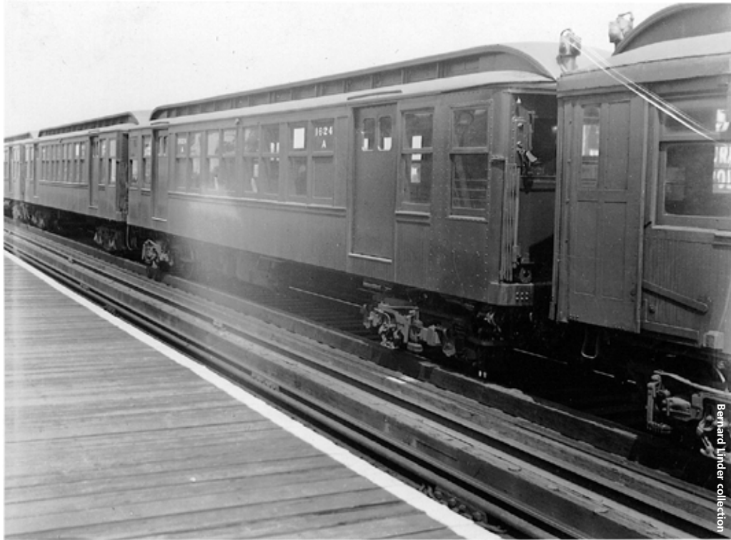
Q-cars with composite car trucks on the Third Avenue "L" at 204 th Street, June 10, 1950.
