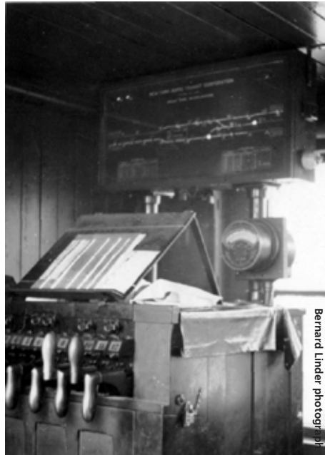
Grant Avenue Tower's interlocking machine.
