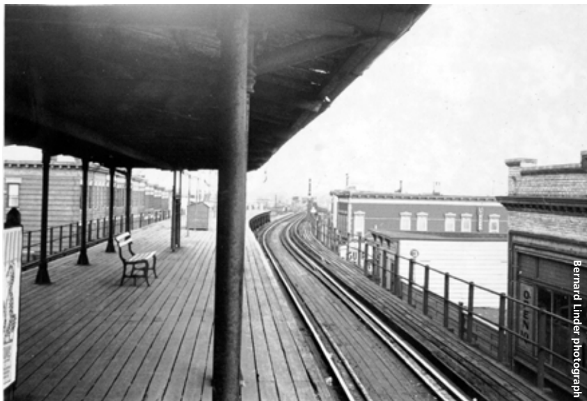
The Grant Avenue station on the Fulton Street "L."
