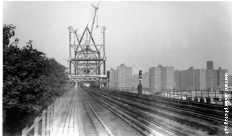
Looking north, toward the third Broadway Bridge under construction, October 11, 1961...
