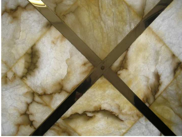
A closer view of the alabaster window in the CREA building (Zaragoza)
