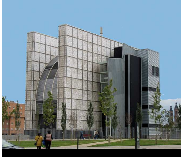
CREA building (Zaragoza)
