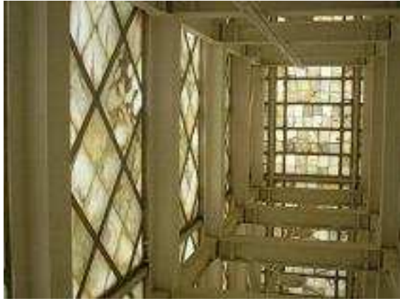
Alabaster walls. A closer view of the inside of the CREA building
