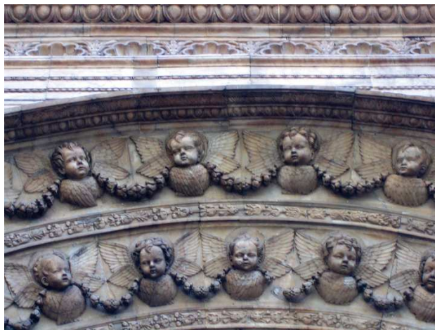
A closer view of the façade in Santa Engracia (Zaragoza)
