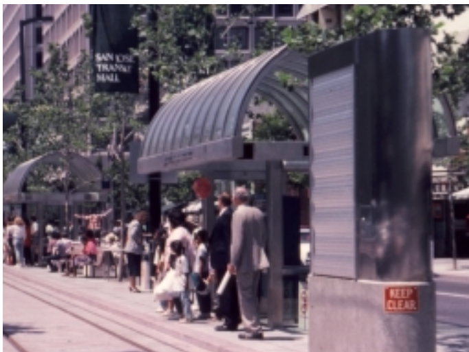
A stationary lift at a station in San Jose.
