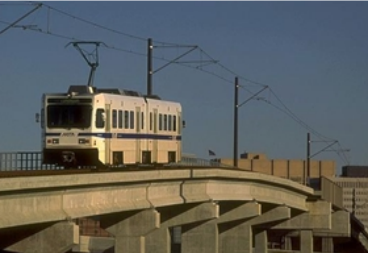
An aerial LRT structure in Baltimore.
