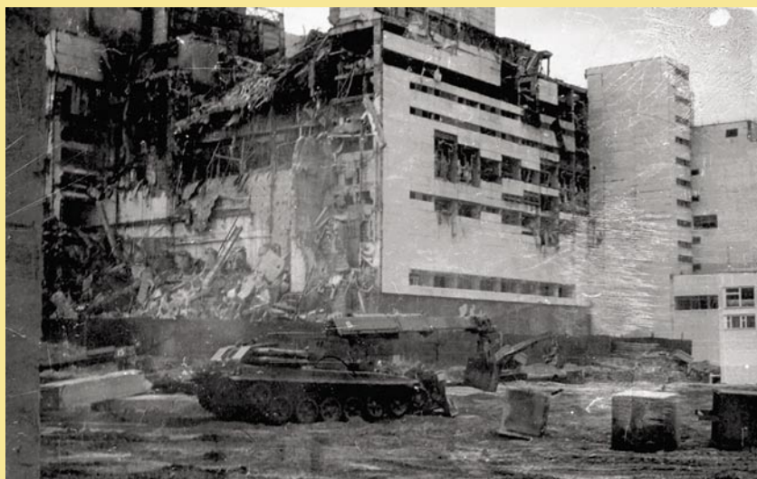
Figure 1: Reactor IV viewed from the north-west, August 1986
