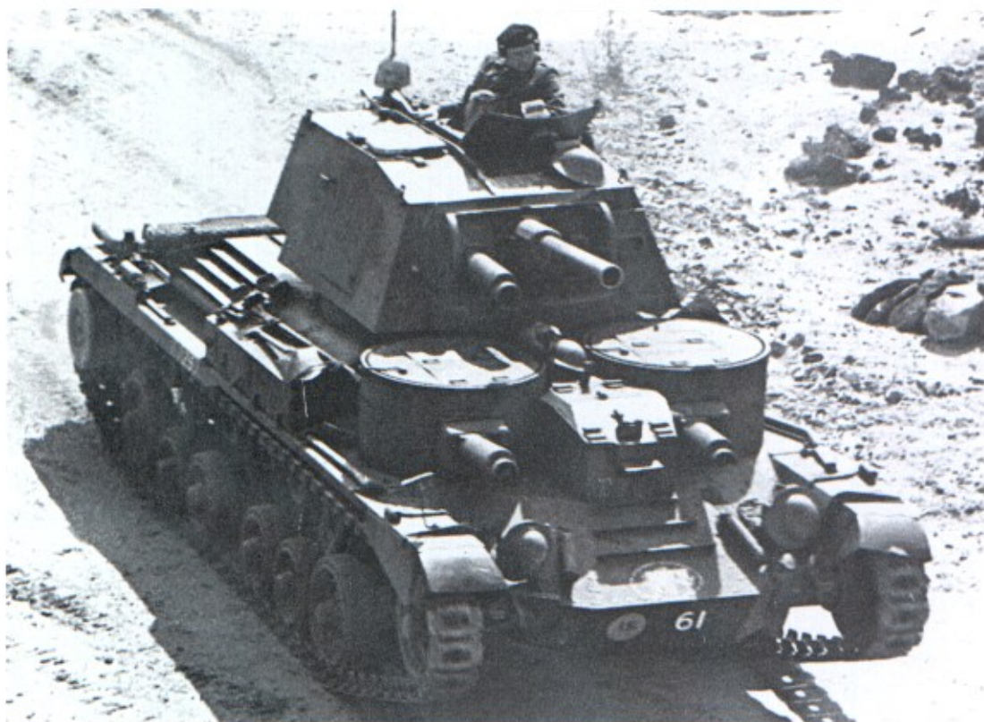
Above: Last of the light tanks - the Light Mk VIII, Harry Hopkins. It was not used on active service, except as the Alecto dozer, there being enough Tetrachs and Locusts for use by the airborne forces. (TM)
