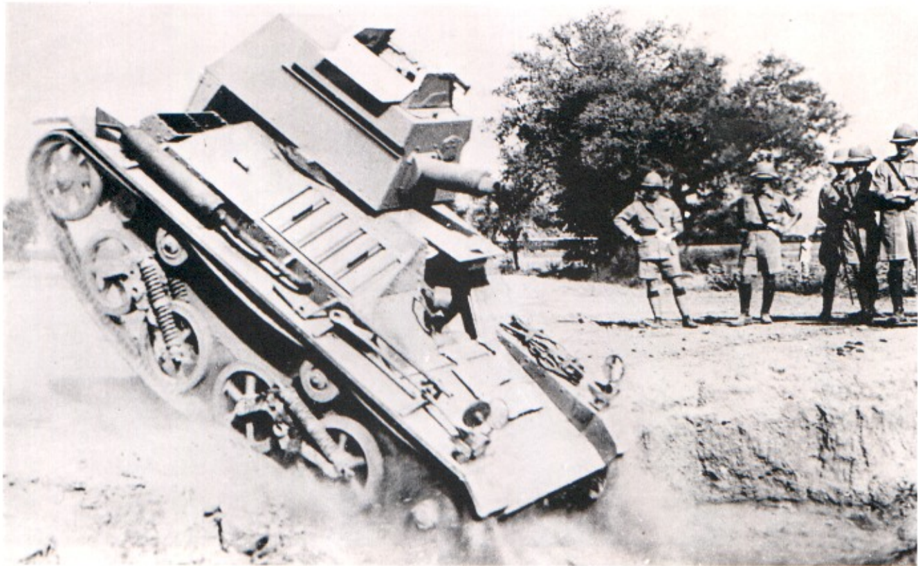
Above: A Light Mk IIB (India pattern) on trials in India, 1935. These little tanks did extremely well, especially over the rough terrain of the North West Frontier. Note the square-shaped non-rotating cupola on top of the turret. (TM)
