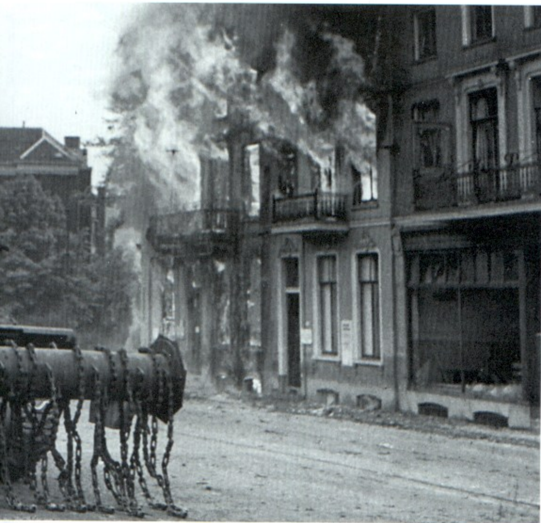
Left: The most successful type of minefield gapping equipment was the British Sherman Crab also operated by US troops. It had forty-three flailing chains on a rotor which beat the ground just ahead of the tank, exploding mines. (TM)
