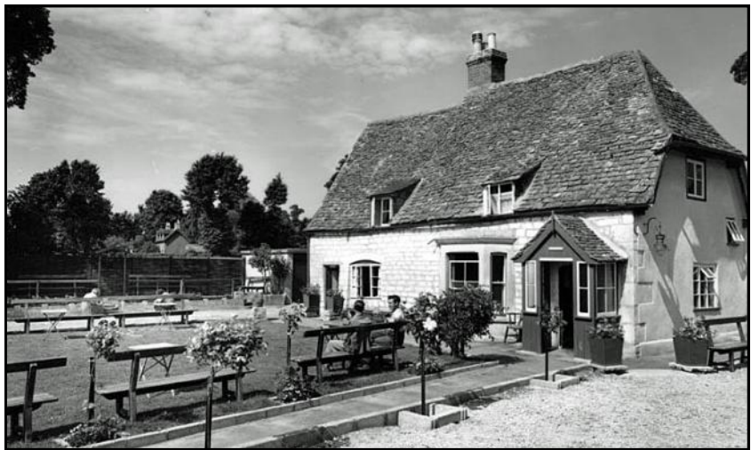
The Spa in the 1950s after refurbishment
