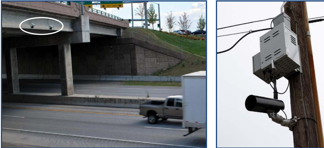
Figure 7: Stationary/Fixed ALPR Cameras on a Bridge and Utility Pole
