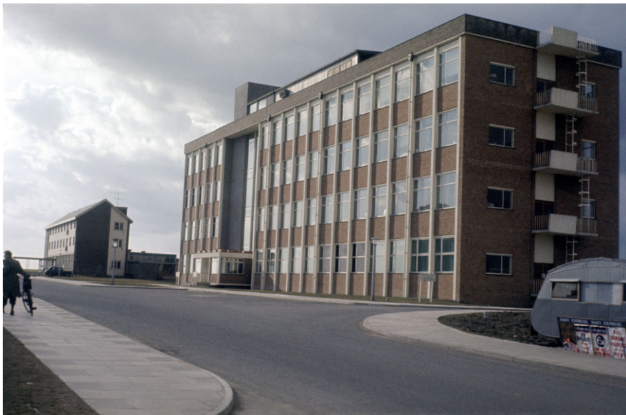
Figure 9. LMB, 1962. The emergency staircase, seen on the right, was replaced with a helical staircase in 1964. (Courtesy of Hans Boye.) (Online version in colour.)
