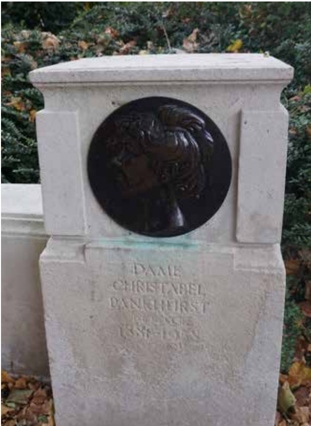
21. Bronze roundel portrait of Christabel Pankhurst by Peter Hills, which was added to the statue in 1959 together with the memorial of the WSPU more generally, and the low curved Portland stone wall, 2017 (Donald Insall Associa
