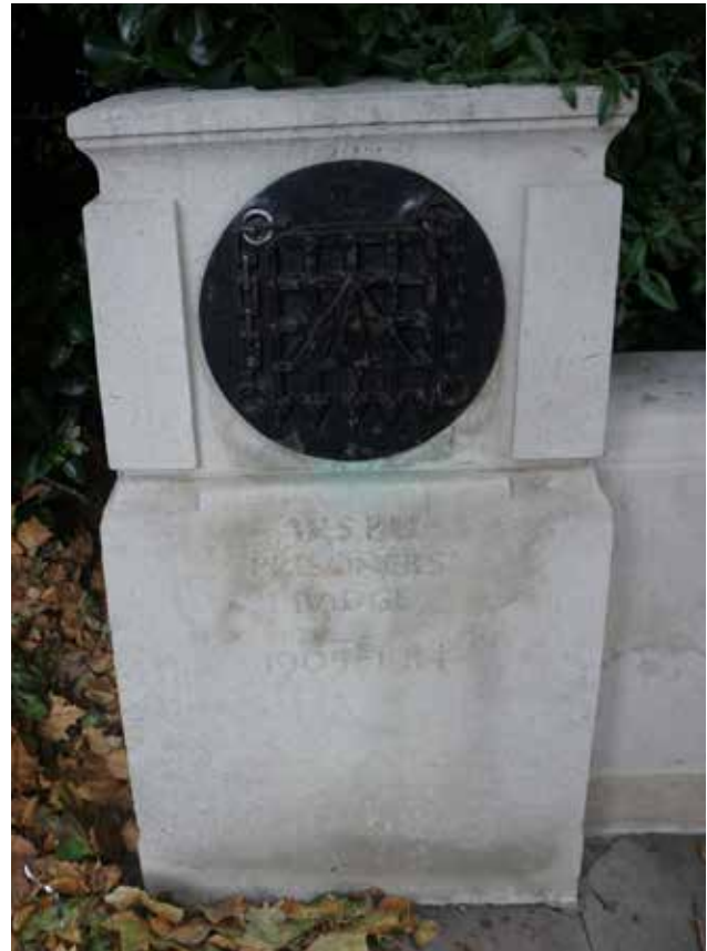
22. Bronze roundel of a WSPU prisoner's badge which was added to the statue in 1959 together with the memorial to Christabel Pankhurst and the low curved Portland stone wall, 2017 (Donald Insall Associates)
