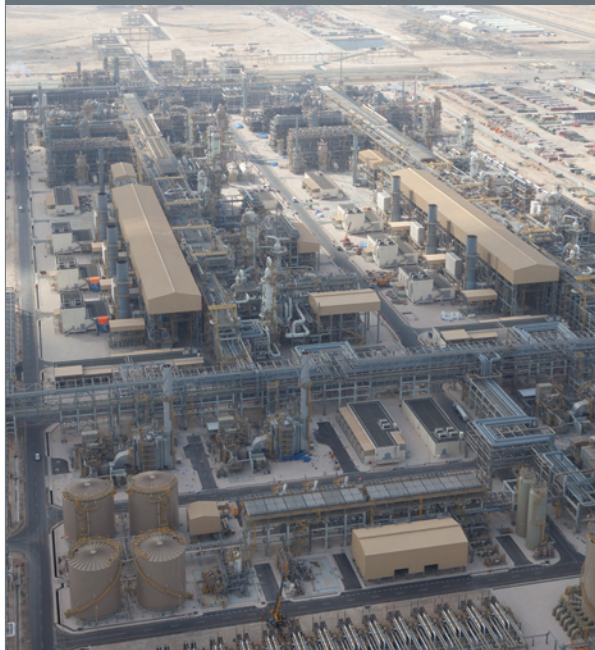
RasGas Trains 6 and 7, over a kilometer in length, are each designed to produce 7.8 million tonnes per year of LNG.
