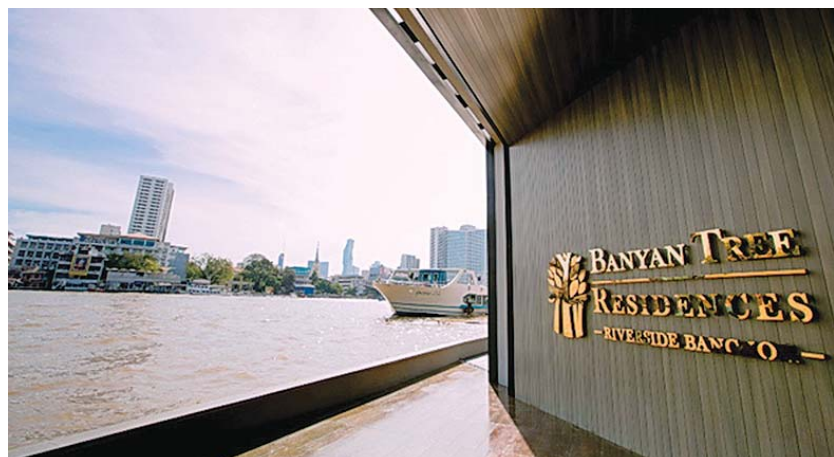
BANYAN TREE RESIDENCES takes shape across the river.
