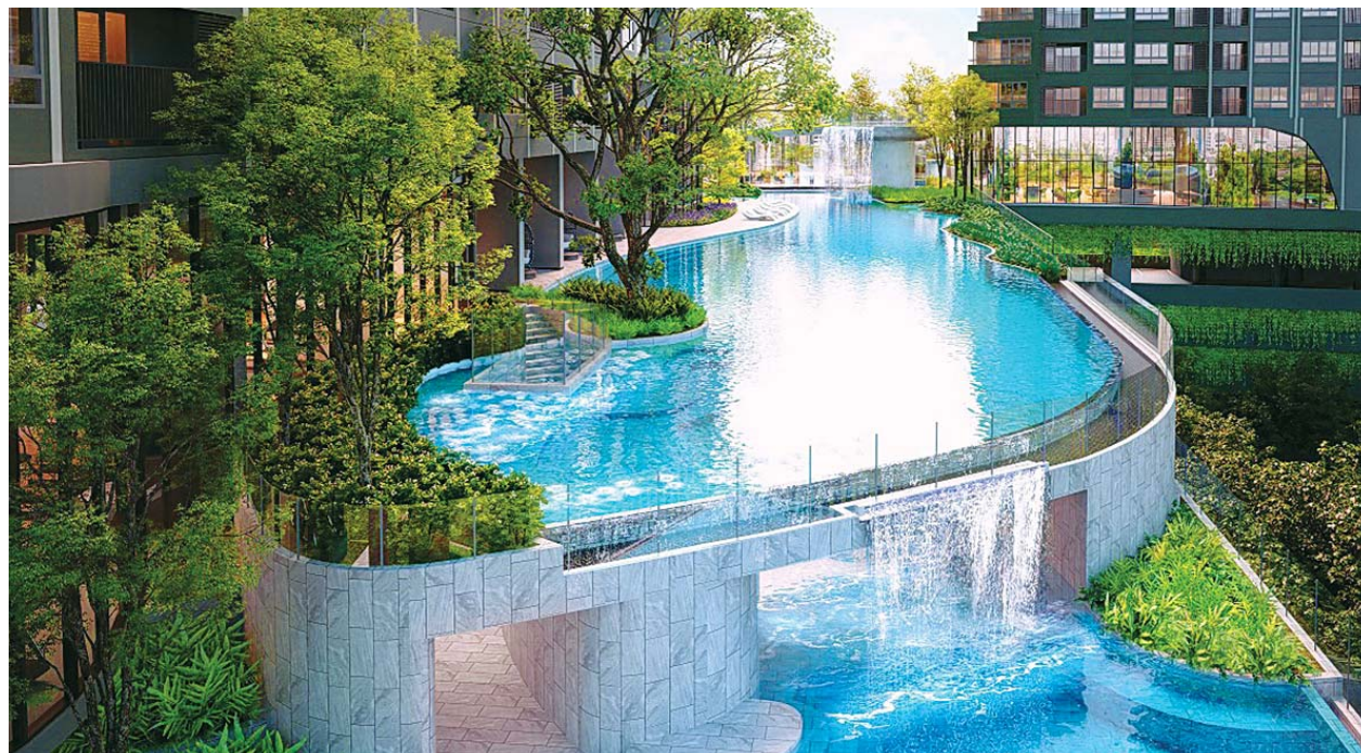
WATER FEATURES AT the new Elio project along the new BTS line.
