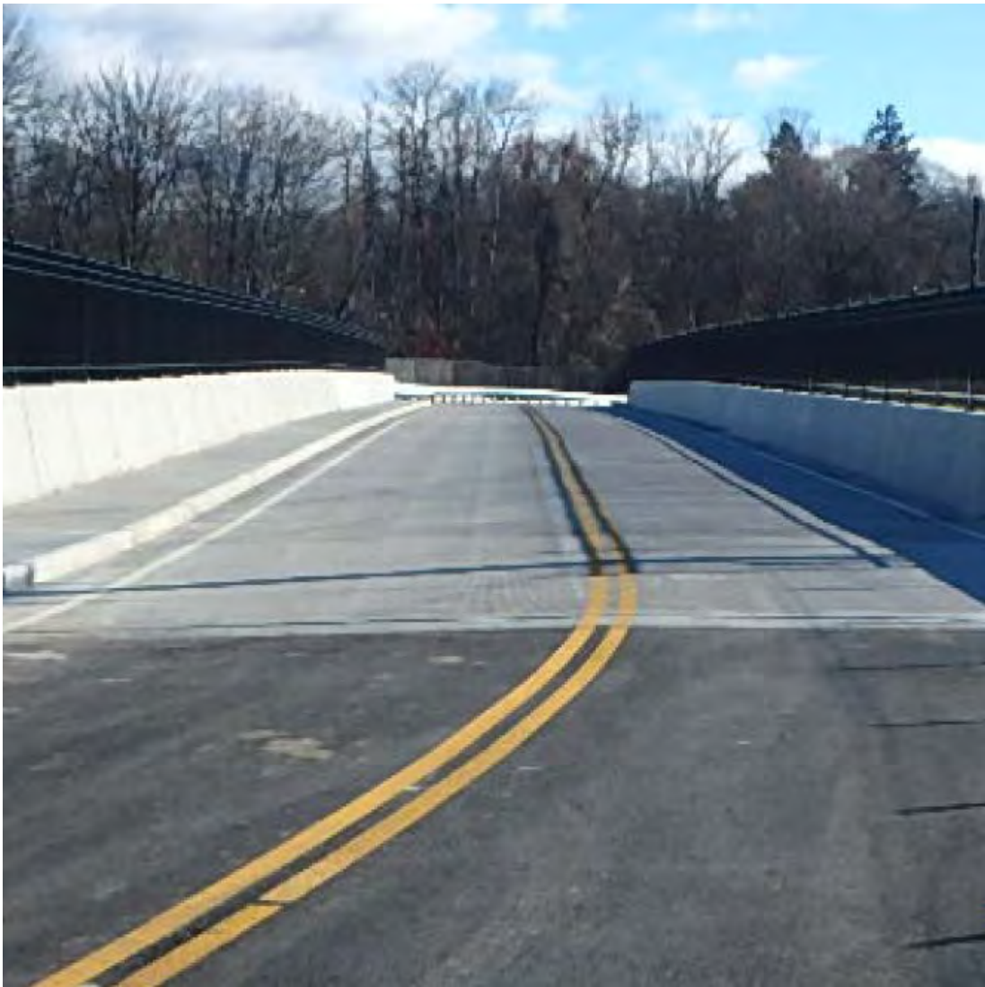
Prospect Hill Road Bridge over Harlem Line and Brewster Yard
