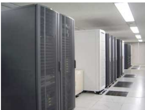
Information Processing Center
