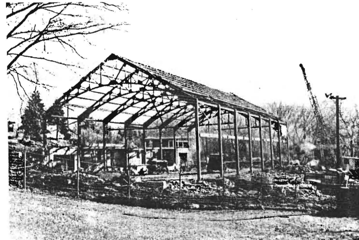
Views of southwest corner of Unit IV during dismantling operations in 1950.
