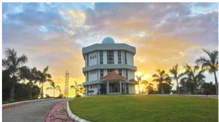
X-band radar building at NARL
