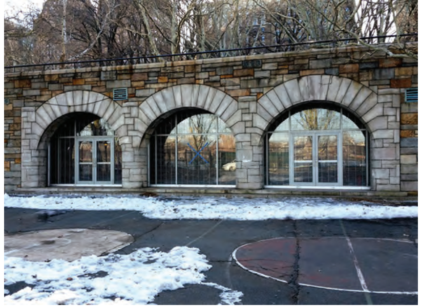
The front of the Field House exterior is now complete.
