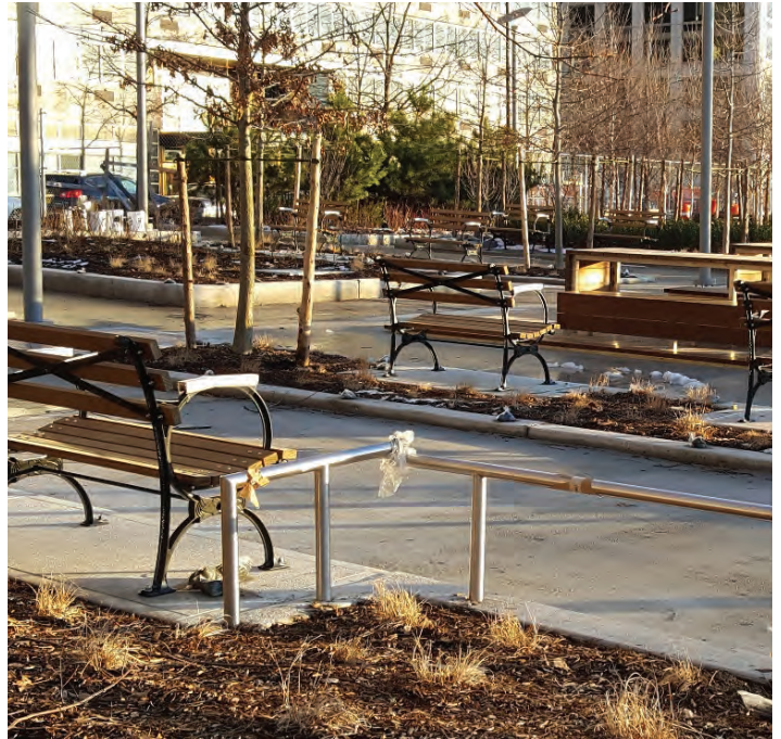
Benches were installed as Phase V work continued in the winter.
