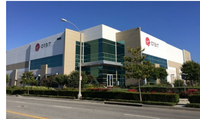
FIGURE 19/ HEADQUARTERS IN LONG BEACH, CALIFORNIA FOR MANUFACTURING AND INTEGRATION
