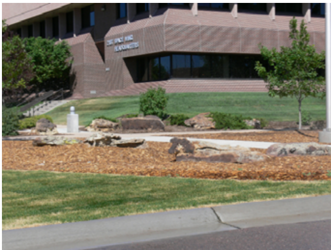
Building 845, Peterson AFB, headquarters of the 21st Space Wing in 2013.
