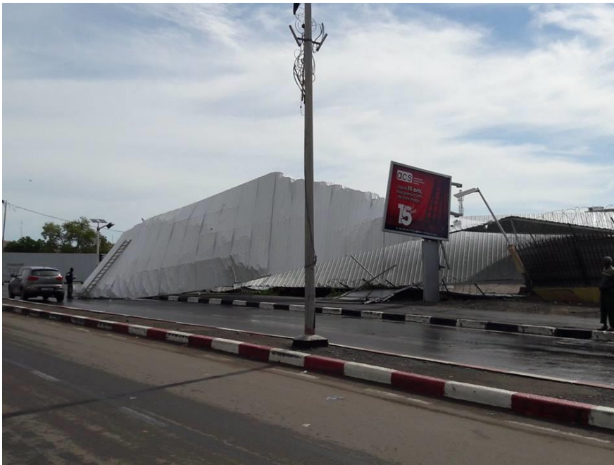
Fig.2.2.9(b) Damage due to CS, Sagar (Source: Djib-Live )
