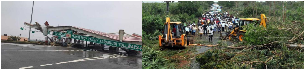
Fig. 2.13.8 (d): Damaged Karaikudi Tollways and blocked roads in Tamil Nadu (The Indian Express 15.11.2018)
