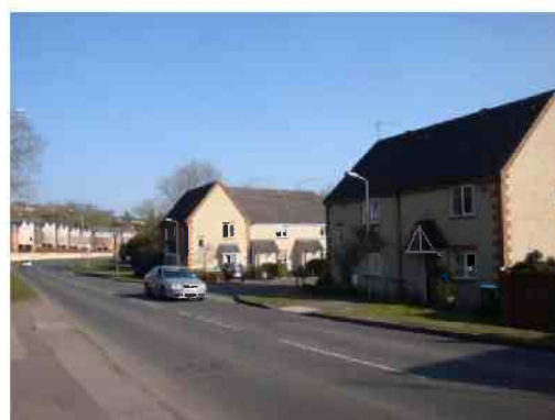
Houses in a depression on Stratford Road, with thresholds below road level
