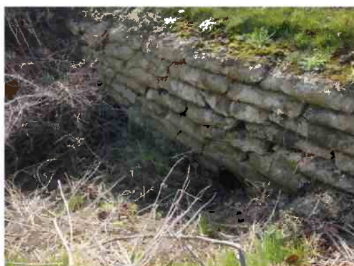
The drainage ditch running along Moreton Road
