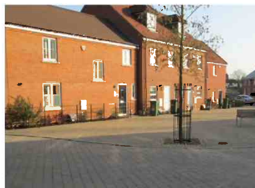
The new housing development off Moreton Road has some areas without kerbs and many houses have very low thresholds
