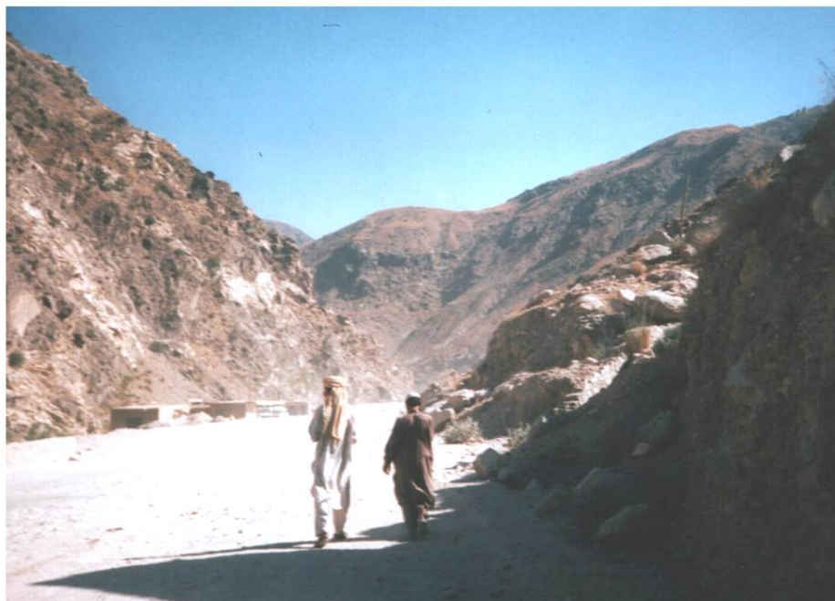
PLATE 7:84, the Road to Kabul, the Jalalabad-Kabul Highway was Literally Destroyed during the Afghan-Soviet War, August 1997.
