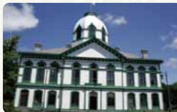
Former Hokkaido Development Commission Sapporo Office Building (reproduction)
