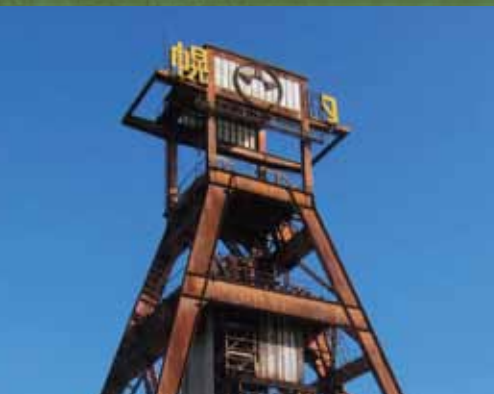
Hokutan Horonai Coal Mine Shaft Tower
