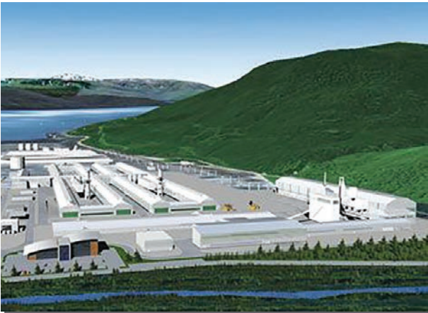
IMPRESSION OF THE $3.5 BILLION ALCAN EXPANSION PROJECT
