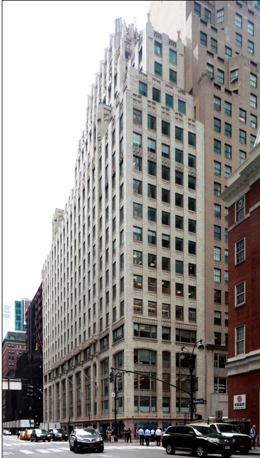
400 Madison Avenue Building Madison Avenue and East 48th Street facades Photo: Sarah Moses, 2016
